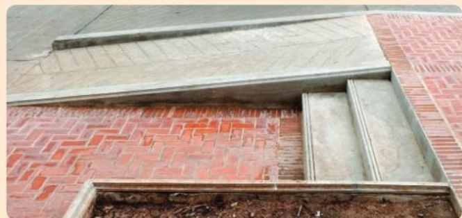
▲ This ramp enables wheelchair access
